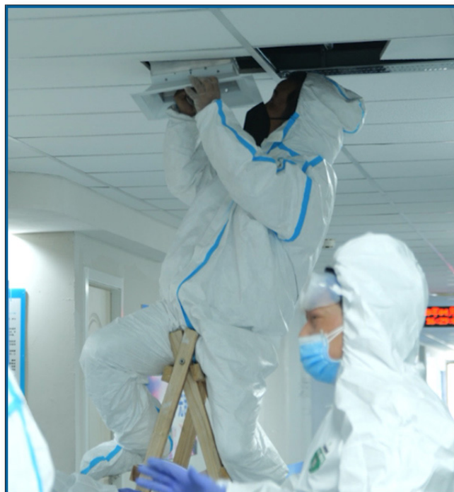
Disinfecting air conditioning ducts.
