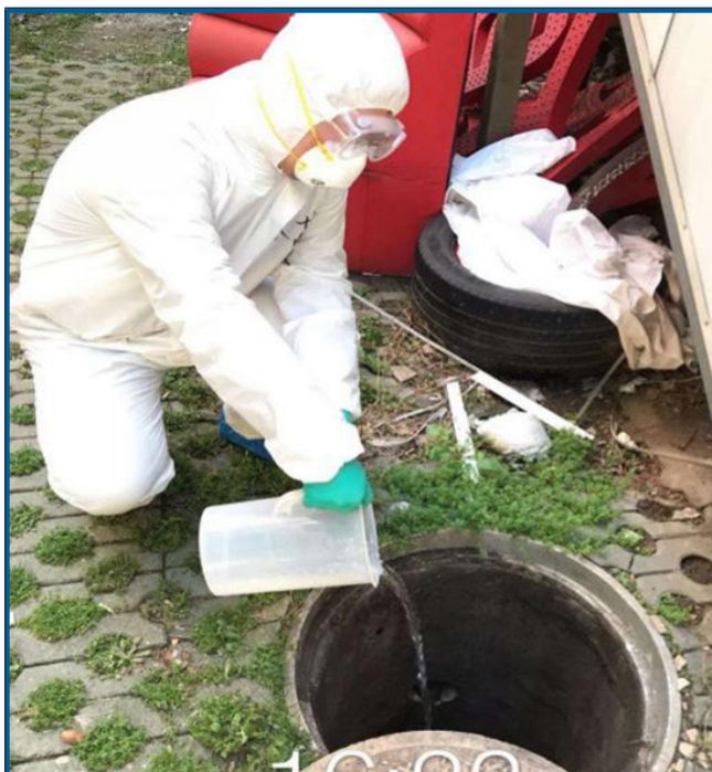
Disinfecting sewage systems.
